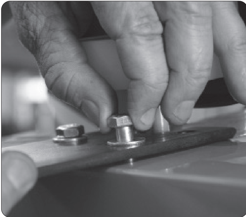
Figure 6 Attaching bracket.
